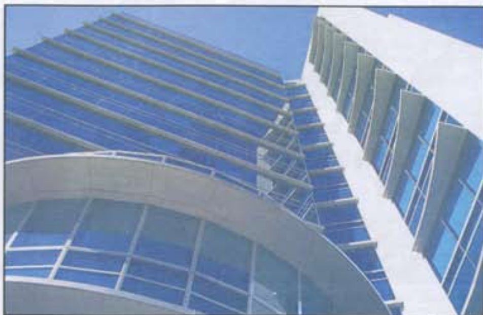
The architect of Qualcomm's 12-story W tower in San Diego, Architects | Delawie Wilkes Rodrigues Barker, is seeking a Leadership in Energy and Environmental Design designation for the project from the U.S. Green Building Council. Photovoltaic panels on the building's parking structure generate power throughout the day to provide lighting to the parking facility at night.
