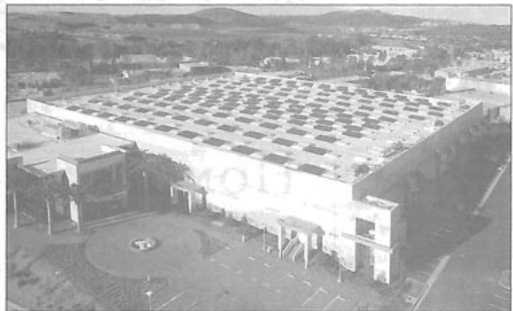
Hunter Industries' new San Marcos facility employs a rooftop photovoltaic system.
