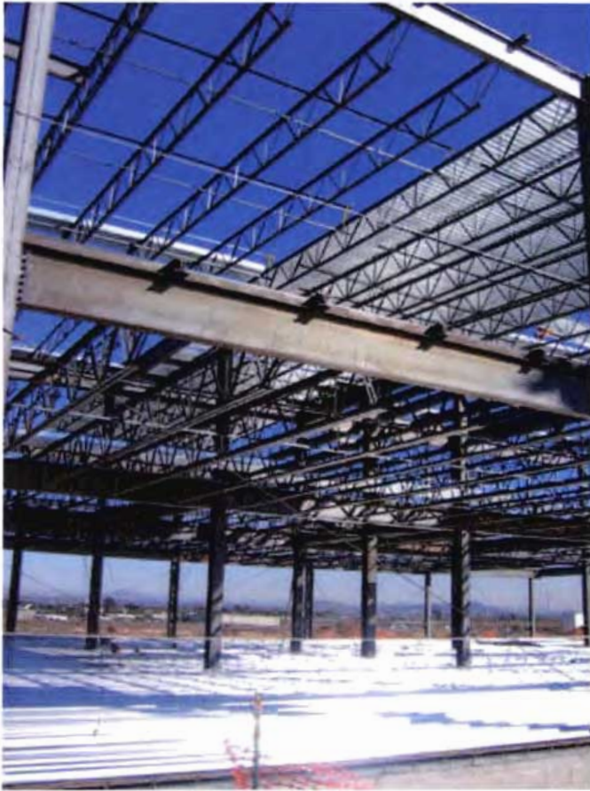
Steel tops out at Bridge Pointe Corporate Centre III
