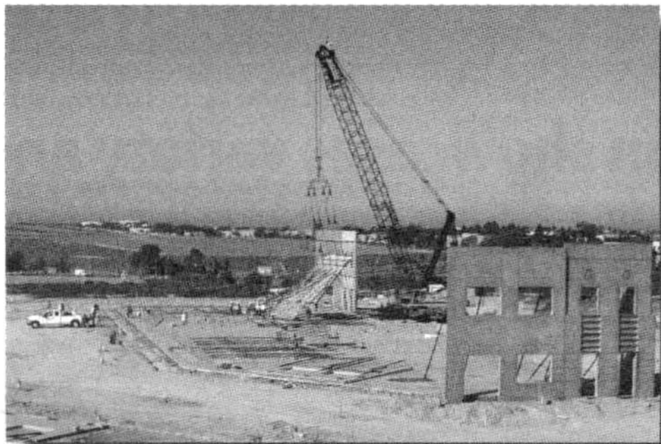
Construction at Bressi Ranch Corporate Center.
